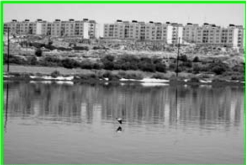
Buildings near the WW ponds affected by Israeli Shelling to the area (Skip 2006)
