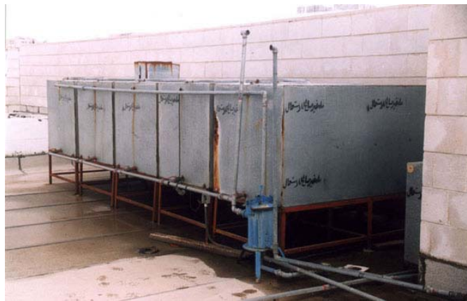
Figure 4.4 King Abdullah Mosque (Photograph by CSBE)
