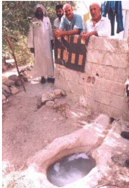
Figure 4.1: Graywater storage in Adasiyyah (Photograph by CSBE)
