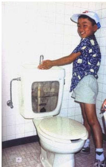
Figure 2.7: Graywater reuse for toilet flushing in Japan (Photograph from Jeppesen and Solley 1994)
