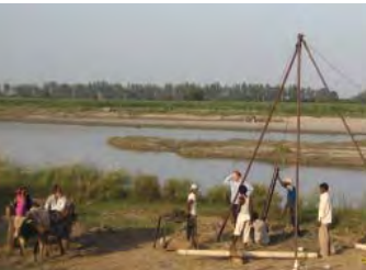
Brunnenbohrung in Delhi Well drilling in Delhi
