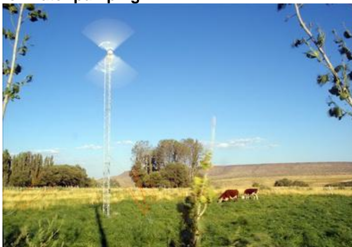
Figure 2.16 A 4.5kW wind energy converter installed in the Michacheo Valley for water pumping
