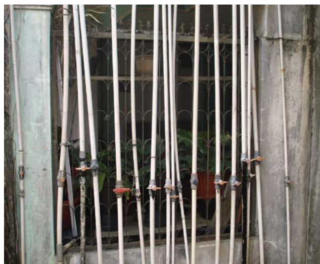
Illegal water connections in Indonesia.
